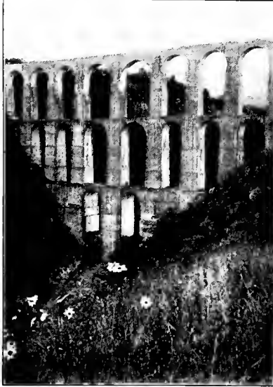
IRRIGATION AQUEDUCT NEAR TEPETZOTLAN Built by Jesuita (XVII or XVIII Century)
