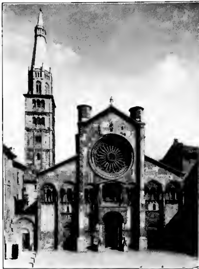
FAÇADE (XII CENTURY), THE CATHEDRAL, MODENA
